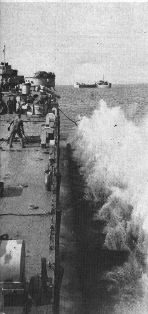
WITH A SPLASH section of causeway is dropped while second waits. Below: LST unloads on Seabee-built causeway.
