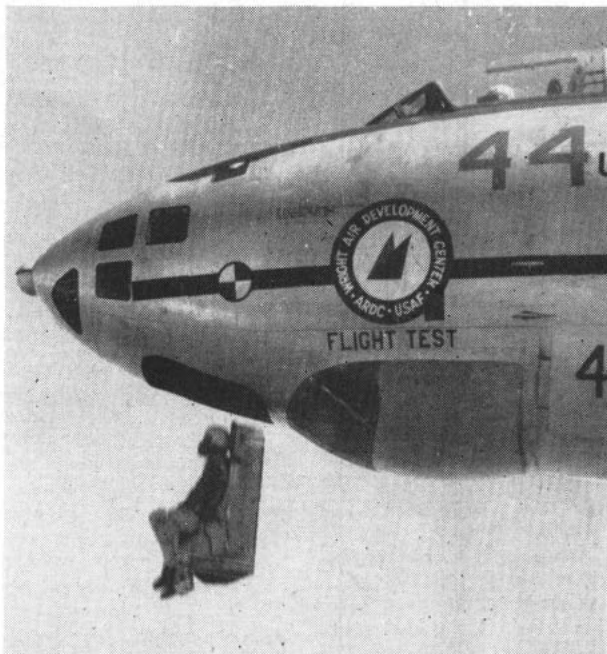
DOWNWARD EJECTION device is used by the Air Force to enable crew members to escape from B-47 jet bomber.
