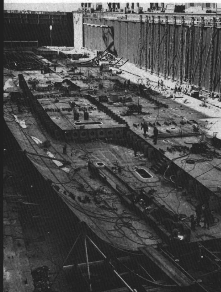
FIRST BOTTOM ASSEMBLY plate for Forrestal was swung into position on July 14, 1952. Below: By January 1953 bottom plates were installed, inner bottoms were begun.
