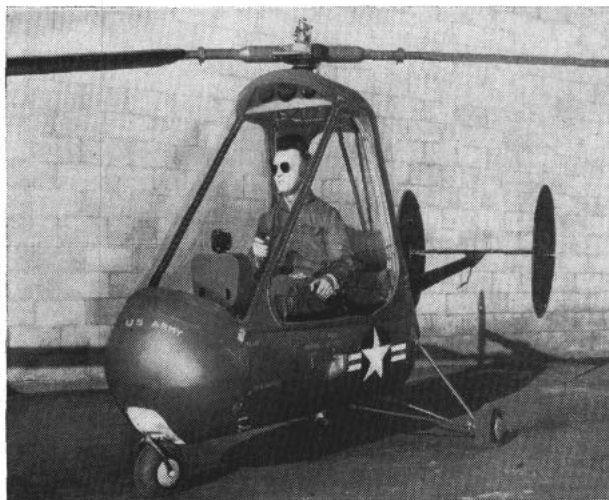
FOR AIR EVACUATION —This small, 330-lb., pulse-jet helicopter can lift two patients in litters attached to its sides.
