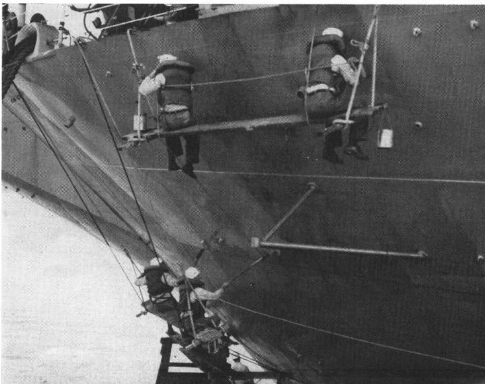
CHIPPING HAMMER and paint are still counted among the leading weapons against corrosion although research is being conducted for new methods.
