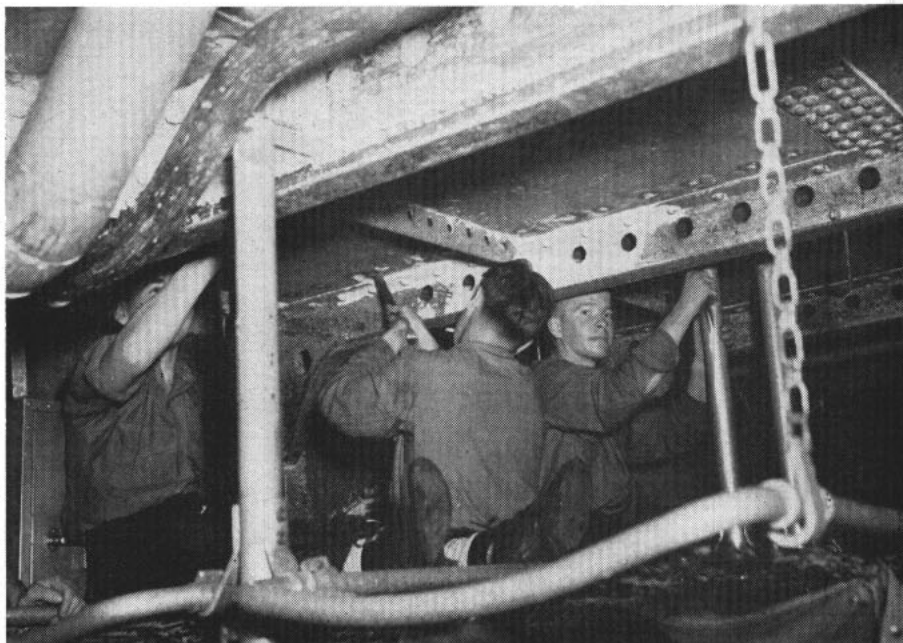
THE SILENT invader is checked by whitehats chipping off old paint: Left: Sand blasting clears the way for protective paints while mothballing ship.
