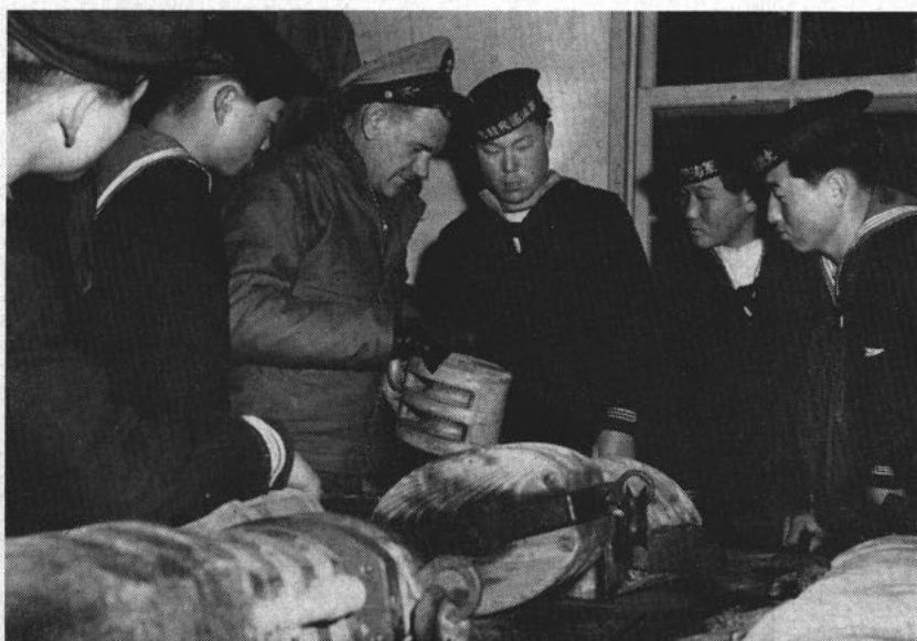
SERVICE SCHOOLS teach all phases of seamanship. Here, Joe E. Brewer, BMC, USN, shows class of ROK sailors the workings of block and tackle.
