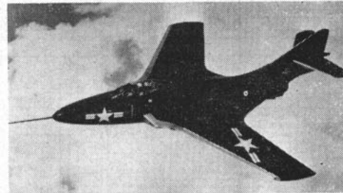
F9F-6 'Cougar'—Swept-wing day fighter, successor to 'Panther,' it is much faster but retains factors making it ideal for carrier operations.
