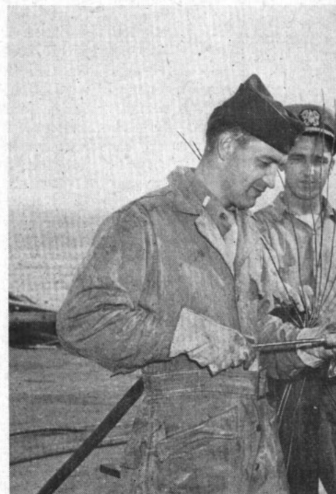
SPlicing of submarine cable which will connect mines to control station on the
