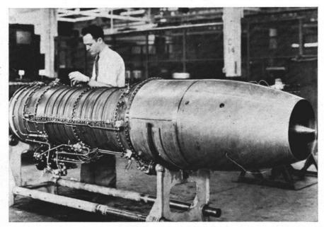
TURBO-JET engine is 24 inches in diameter and is mounted in wing roots. Air streams from the engine's tail pipe at approximately twice the speed of sound.
