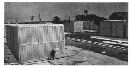
STORAGE cells (above) have vapor-tight access doors. Interior view (below) shows plane and small bags of a desiccant which absorbs water from the air.
