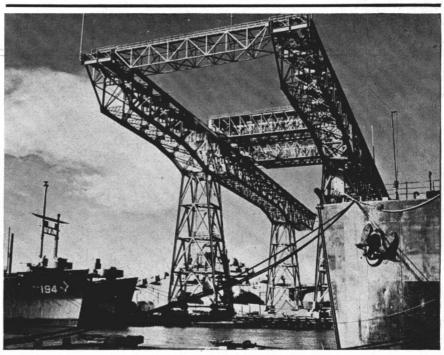
WORLD'S largest crane being completed by the Navy will permit speedier repair of major fleet units. Operators will talk to ground crews by two-way radio.
