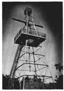
LIVE fuzes mounted in bombs receive drop-tests daily from 75-foot drop-tower situated at Naval Ordnance Lab.
