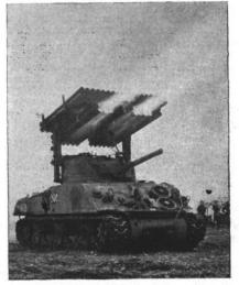
Official U. S. Army Signal Corps photograph ROCKET TANK, revealed publicly last month, helped blast Army's way into the heart of Germany.
