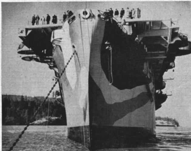
**FOR THE BRITISH:** *The HMS "Tracker," an aircraft carrier made by converting the hull of a cargo ship, made a trial run off Pacific coast . . .*
