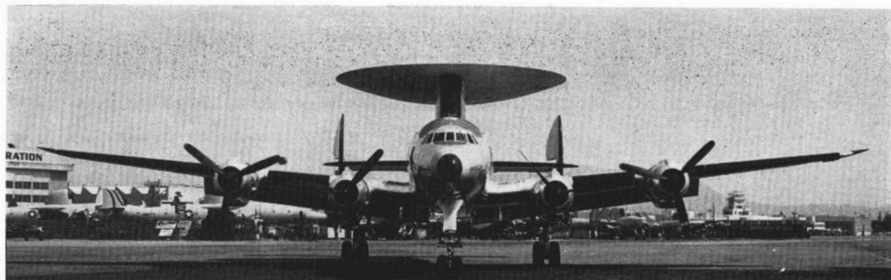
FLAT HAT—Navy's new early warning research plane with 30-foot ellipsoid 'saucer' will test AEW ideas.
