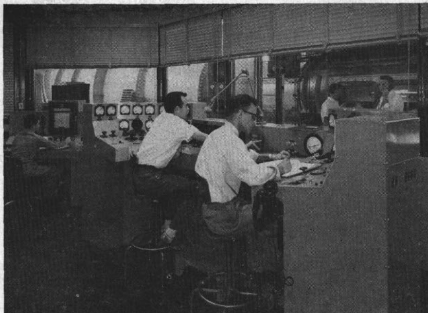
MEN in background observe tunnel and relay data or suggest changing water speed, temperature, etc., to technicians in control console section.
