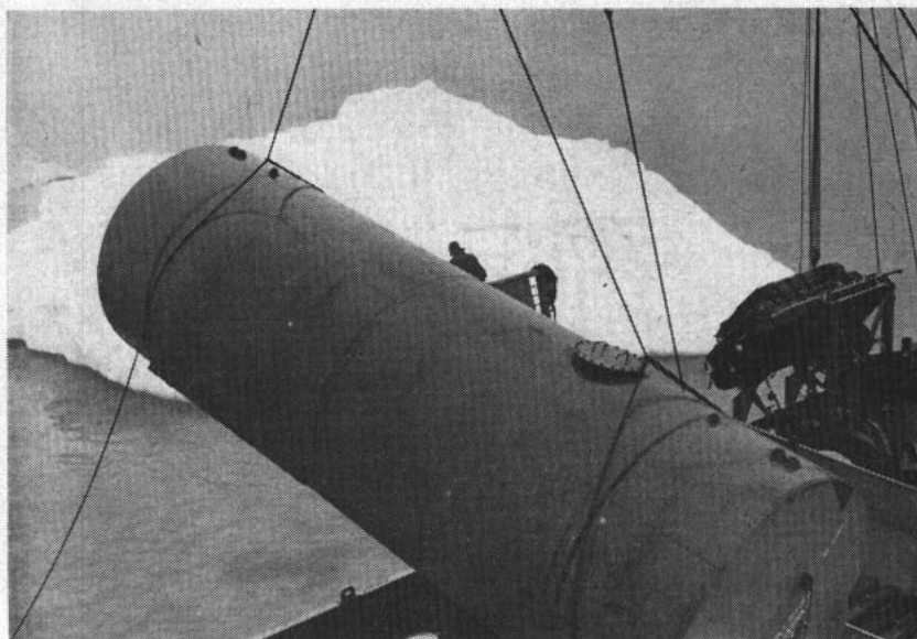
FUEL STORAGE TANK is unloaded from USS Achernar (AKA 53). Tanks like this are used to store fuel on the base. LSMs carry tanks from ship to shore.
