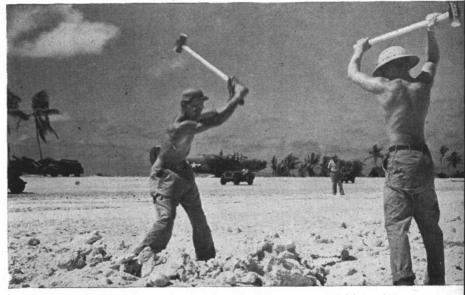
SEABEES attached to Acorns have job of building new airfields and improving and repairing captured fields. Husky Seabees (above) pound coral lumps into sand for Eniwetok runway. Another airstrip (below) is built of metal mats.
