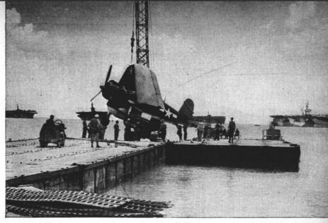
EMBALMED planes were taken to the Marshalls by jeep aircraft carriers, ferried ashore by outboard-motored pontoon barges. Here one of the planes is hoisted to pontoon dock where tractor waits to tow it to assembly line.
